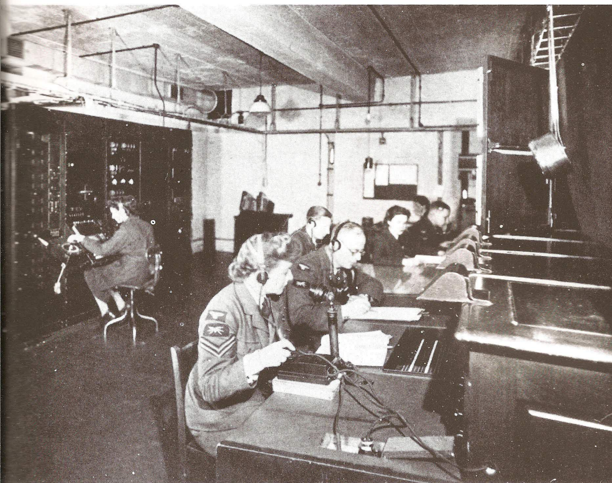
Fig. 14. CH receiver room
