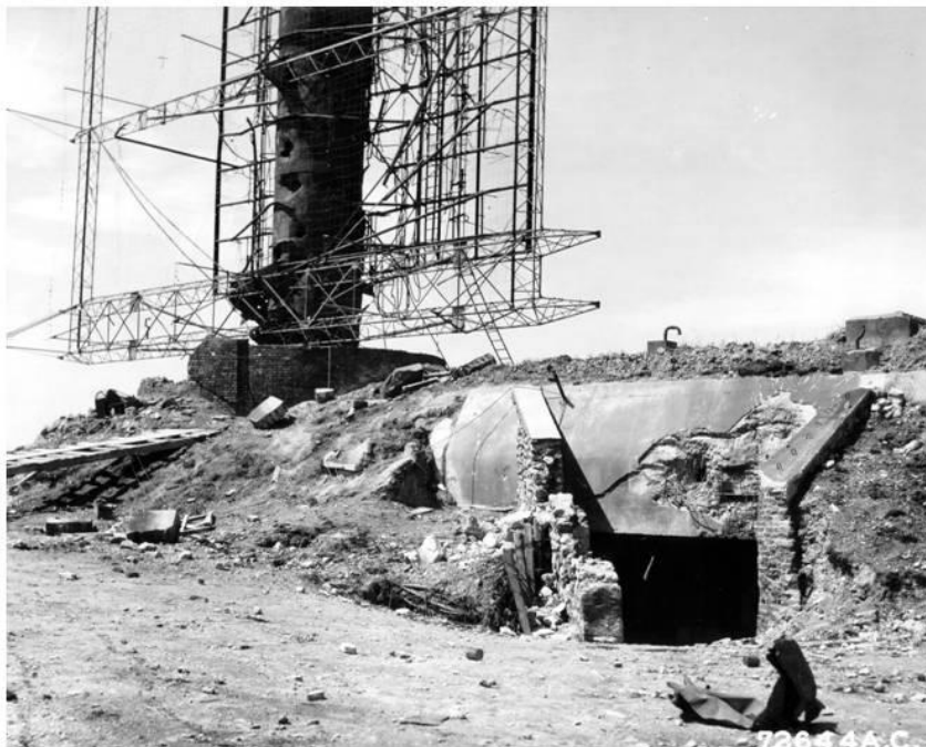
Figure 8. The Klein Heidelberg at TAUSENDFÜSSLER (Cherbourg). In this installation the Wassermann-S antenna was retained on the rear side of the KH array. In both pictures, but particularly the lower one, substantial damage is evident to the antenna, the tower and the bunker (Conseil Régional de Basse-Normandie / US National Archives).
