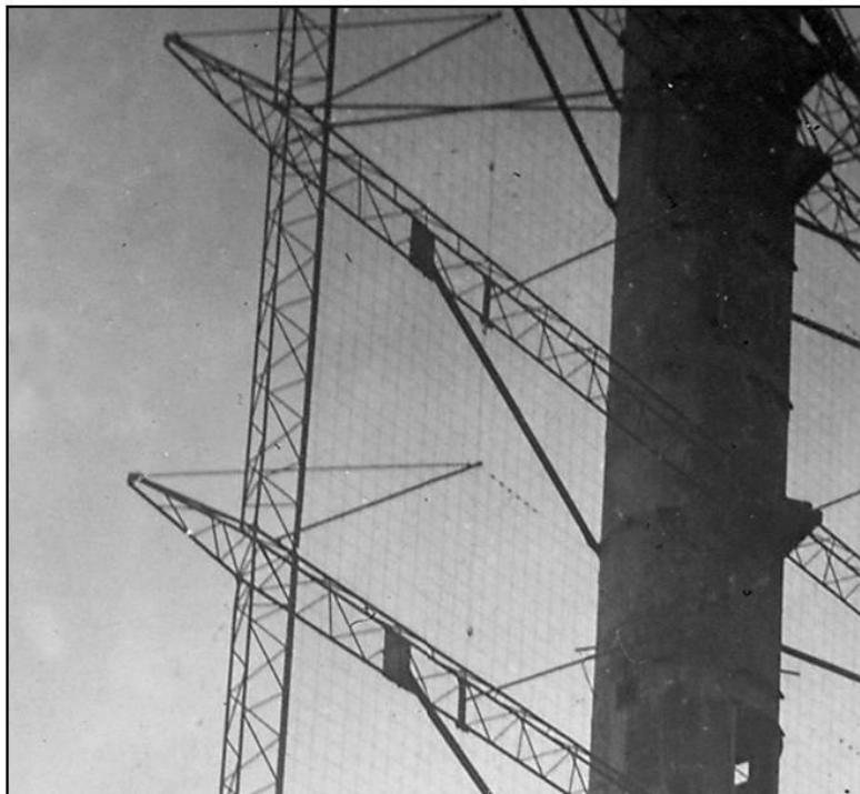
Figure 9. The second Klein Heidelberg, at BIBER (Oostvoorne). In this installation the Wassermann-S antenna is absent. The lower picture shows an expanded view in which the dipole elements and the wire mesh reflector are visible (© Jeroen Rijpsma).
