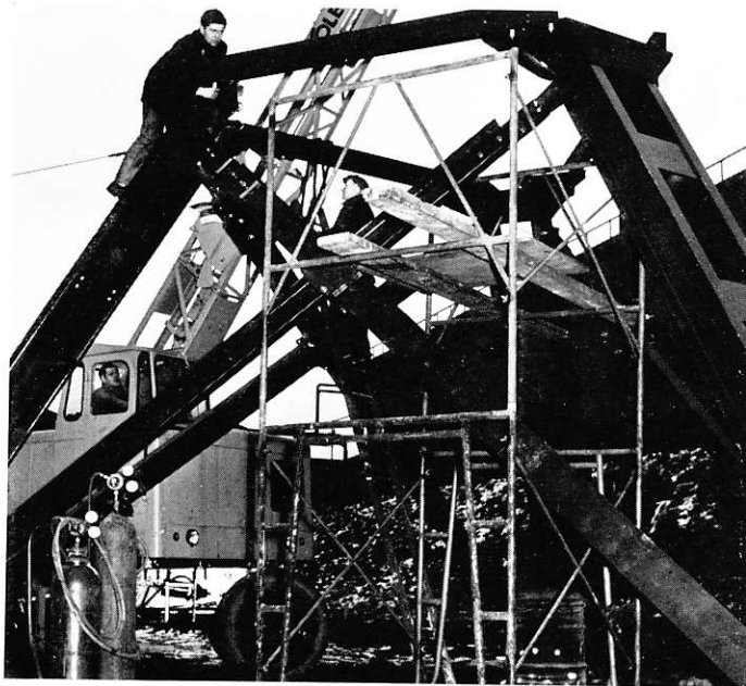
ABOVE: A gantry for the Apollo dish aerial being erected for test at Felling Works before being sent to Rivenhall. Driving the crane is G. Rutter, Felling Transport, and the fitters are A. Yeaman, left, and W. Bell [Turner's, Newcastle]
