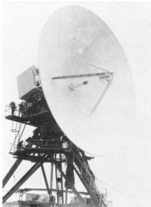
Almost complete. The aerial on its mounting showing the feed horn, and the rotating sub-reflector held by the tripod fixture. The transmitter moves with the aerial
