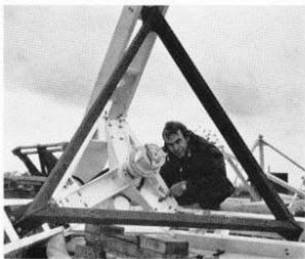
A mechanical engineer working for Space Communications Division, David Oliver works on the sub-reflector mounting just before it is hauled into position by the crane
