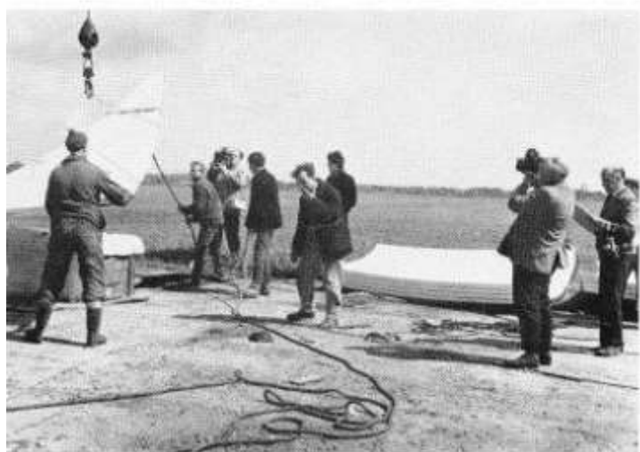
Working in a 40 m.p.h. wind with a sprinkling of sleet and hail, the Rivenhall riggers hoist the 'petals' for the aerial. A steady rope is held by Brian Marjoram
