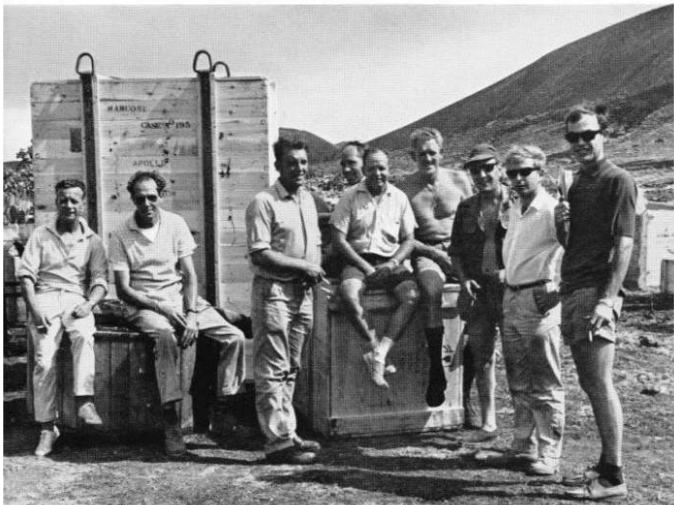
The aerial-erection team—engineers and riggers. Left to right: Johnnie Thompson; Doug Clements; Peter Bowkett; Frank Quinn; Monroe, the American crane-driver; Harry Wilson; Billy Ash; Brian Marjoram, and David Oliver
