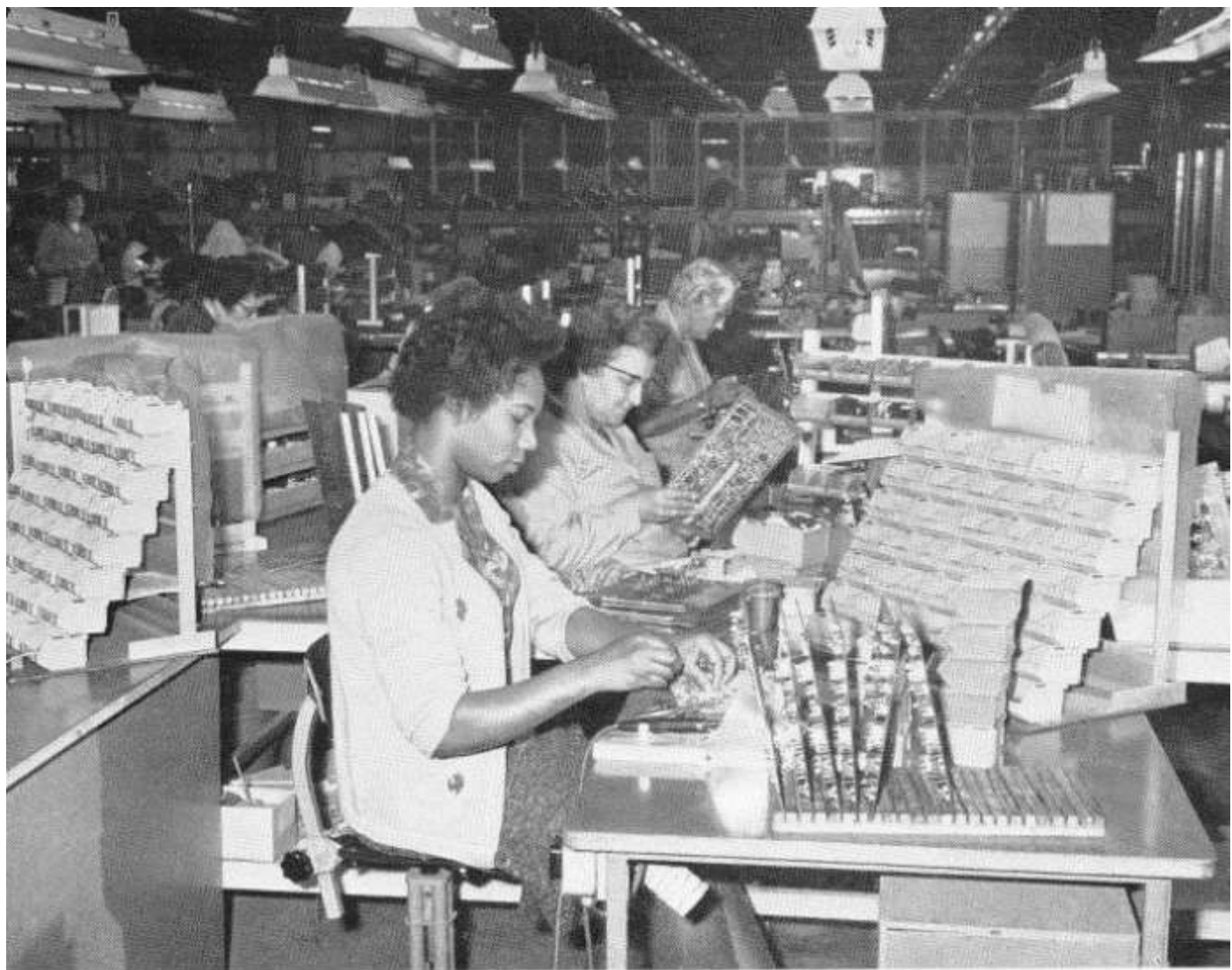
These pictures show the new layout of the benches and supply racks. ABOVE: Circuits being assembled for H2000 MST communications receivers, which are being sold all over the world, some to NATO. The girls position the components by the numbers on the plan and tack them in with solder. Left to right, Mrs. Doxie James, from Jamaica, Gwen Cox and Mrs. Ruby Freeman. BELOW, LEFT: Mrs. Hazel Bailey, centre, who also operates the flow-soldering machine which completes the joints. To the left, behind, is Mrs. VI Rees, and right, Mrs. Irene Blake. BELOW, RIGHT: Mrs. Cora Porteous at work on H2000 circuits
