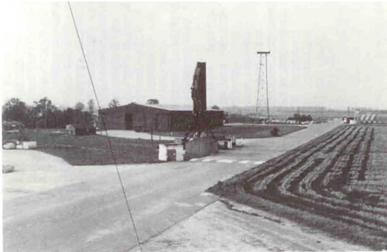
Type T2 hangar on the West side of the airfield, used for radar assembly and testing and much modified by GEC Marconi in the 1960's.
