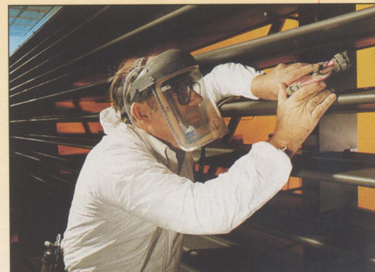
RIGHT: Paint spraying.
