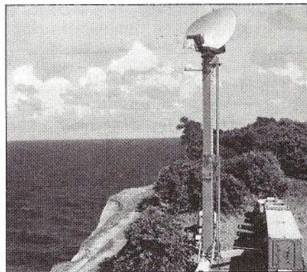
Figure L2. S-band low cover radar type S711 on a 60 foot telescopic tower.
