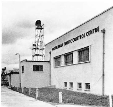
The aerial of the radar link transmitter was mounted on a temporary tower at the Southern Air Traffic Control Centre, London Airport. Signals from the radar and from the television O.B. van were carried by cable to the link transmitter which was specially installed in the equipment room at S.A.T.T.C.
