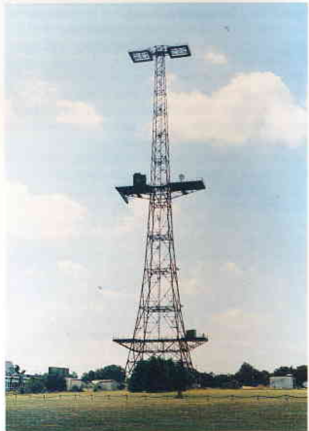
3 A CH transmitter tower, formerly located on the Essex coast at Canewdon, now at the GEC-Marconi Research Centre, Great Baddow.
