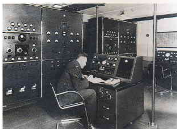
7 East coast CH transmitter room
