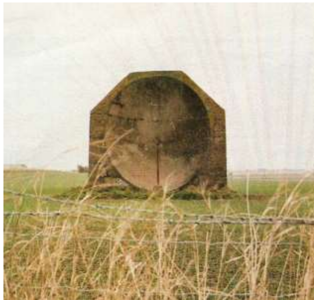
Figure 9. Concrete WW1 sound locator at Kilnsea, Yorkshire (Author's collection).
