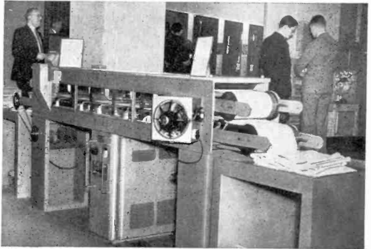
Typical applications of the Redifon RH7, 2-kW radio heater. (Left) Gluing sixteen joints simultaneously in 3 minutes in a hydraulically operated jig and (above) conveyor for drying textiles and similar materials.
