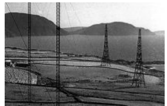
Chain Home Dalby in 1949 – metal lattice transmitter masts on the left, wooden receiving-aerial towers on the right (John C Hall)
