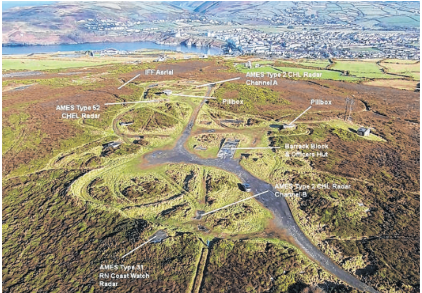
Location of WWII radar installations on Meayll Hill
