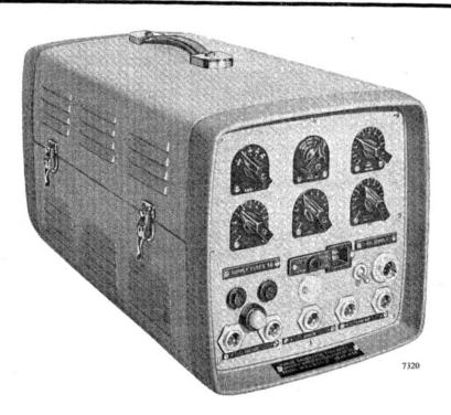
THE FUNCTION of the Radar Range Calibrator, Type SI 101, is to facilitate the accurate testing of range calibration and thereby the linearity of timebase circuits with reference to crystal standards.
