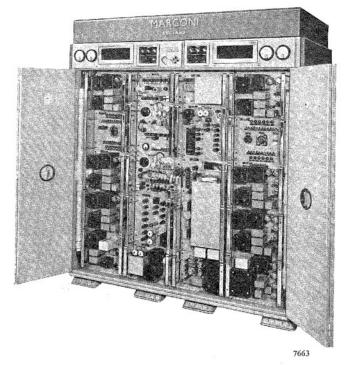
either side of it. The cabinet doors enclose these gates and full protective interlocks are incorporated. No rear access is required.
