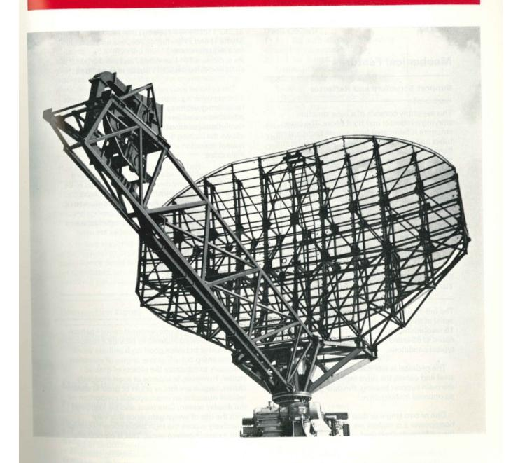
Double-beam aerial for enhanced target to clutter ratio
