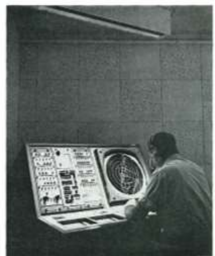
A typical display position with selection of SSR facilities
