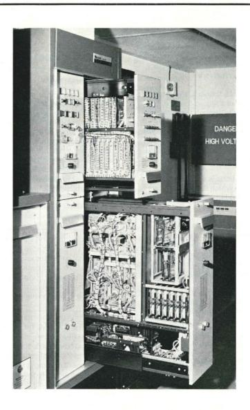
Complete heightfinder aerial control, using solid state components
